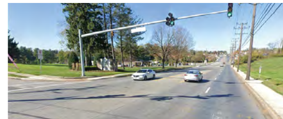
Lack of pedestrian crossing infrastructure and narrow, unbuffered sidewalk on arterial roadway in Pikesville.
