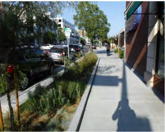
Incorporating green infrastructure, such as the bioswale pictured above, helps manage stormwater and runoff and improve the walking and biking experience.
