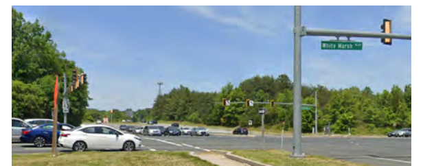
Major intersection at MD-43 and White Marsh Blvd with pedestrian crossing signals missing from some crossing legs.
