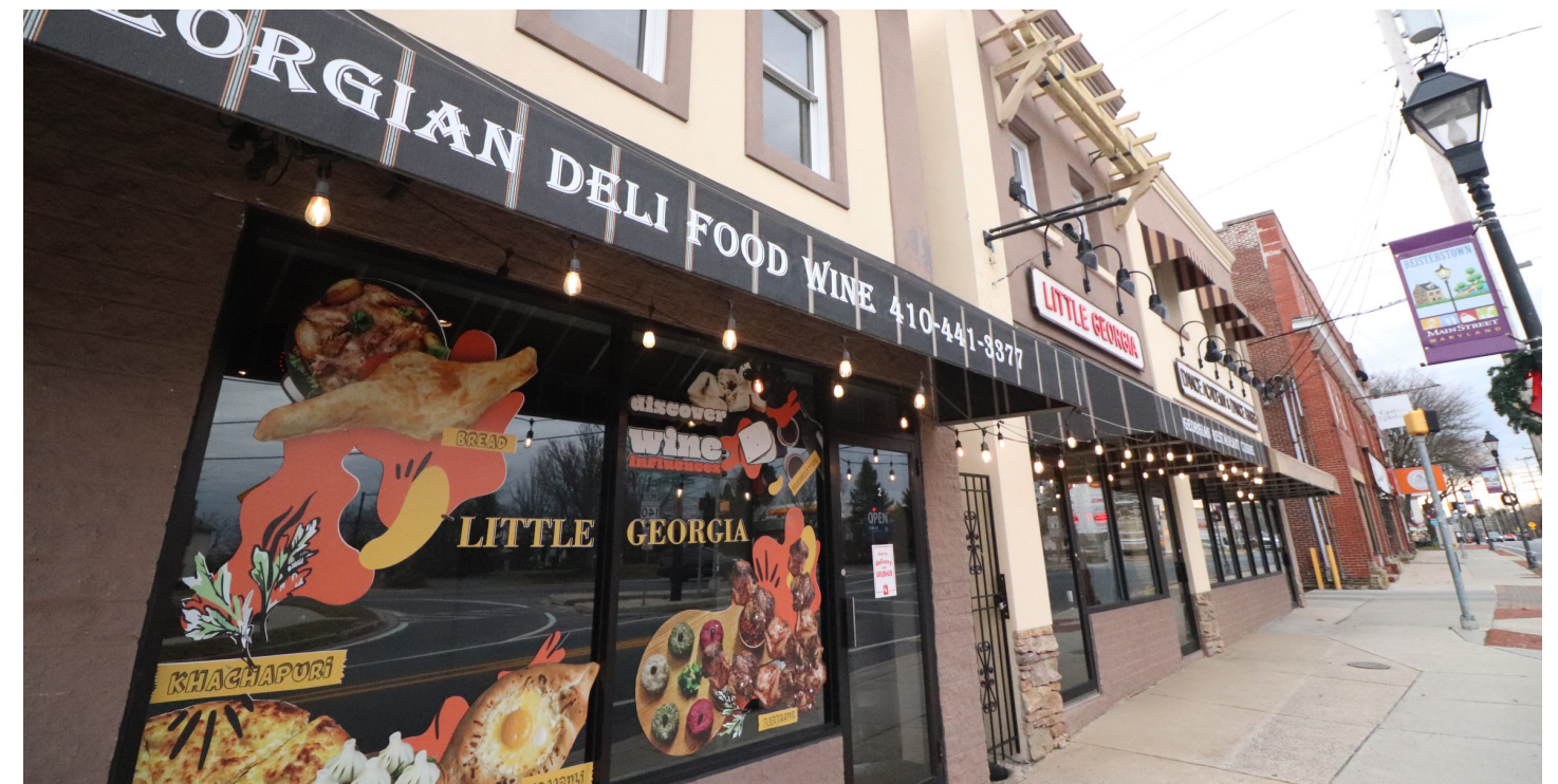
Businesses using architectural elements such as overhangs, awnings, lighting and interesting signage to create a visually appealing facade and streetscape. (Existing facades from Reisterstown Road).
