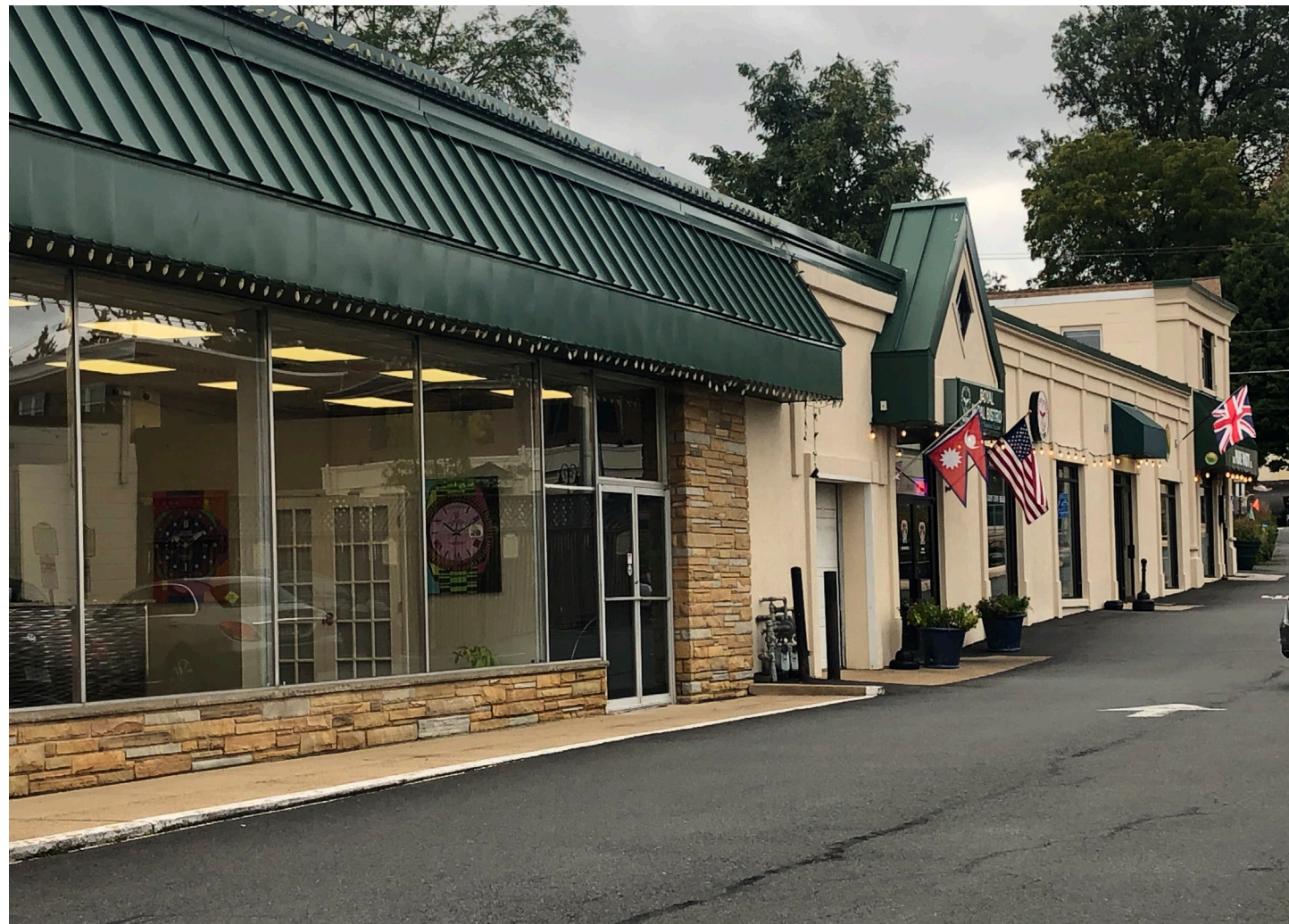
Awnings, roofline shape and height changes, architectural detail, and materials break up the continuous facade into storefronts. Image courtesy of NDC.
