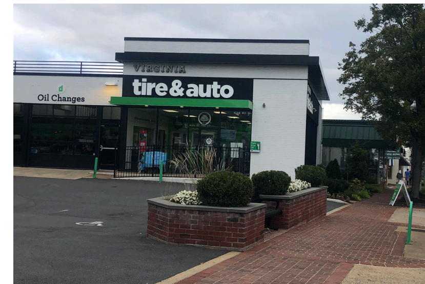
Masonry planters screening a parking lot and delineating public sidewalk
