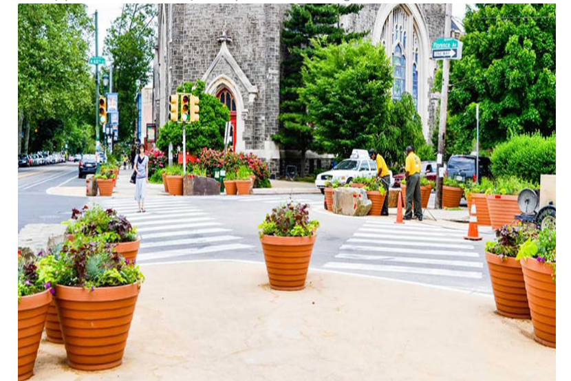
Philadelphia pedestrian improvements using painted bump outs and planters
